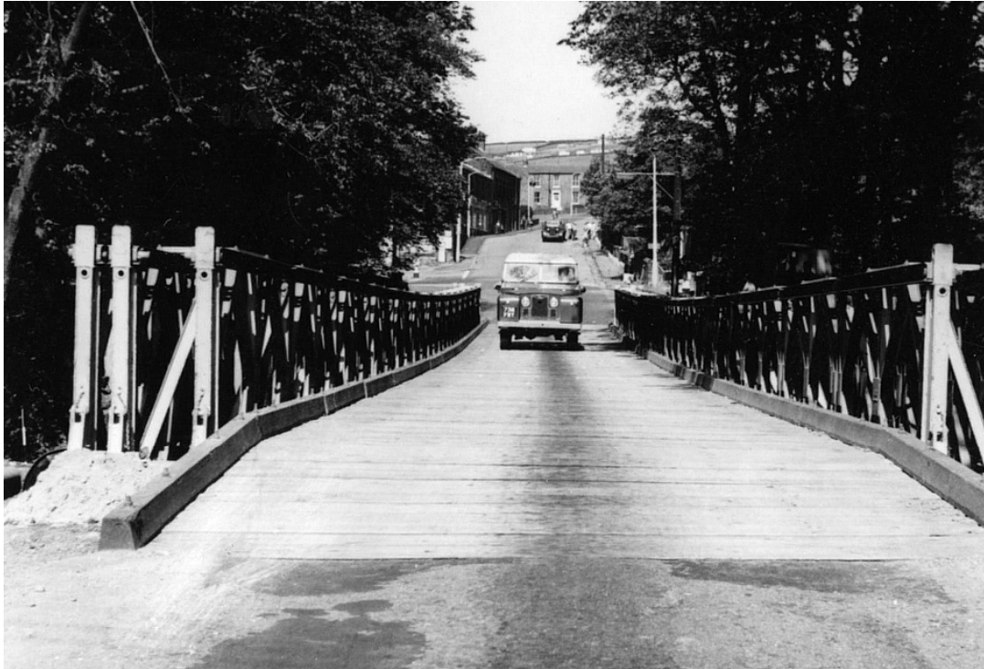
Figure 11. The Bailey Bridge over the Collapsed Culvert - Denshaw, 1964.
