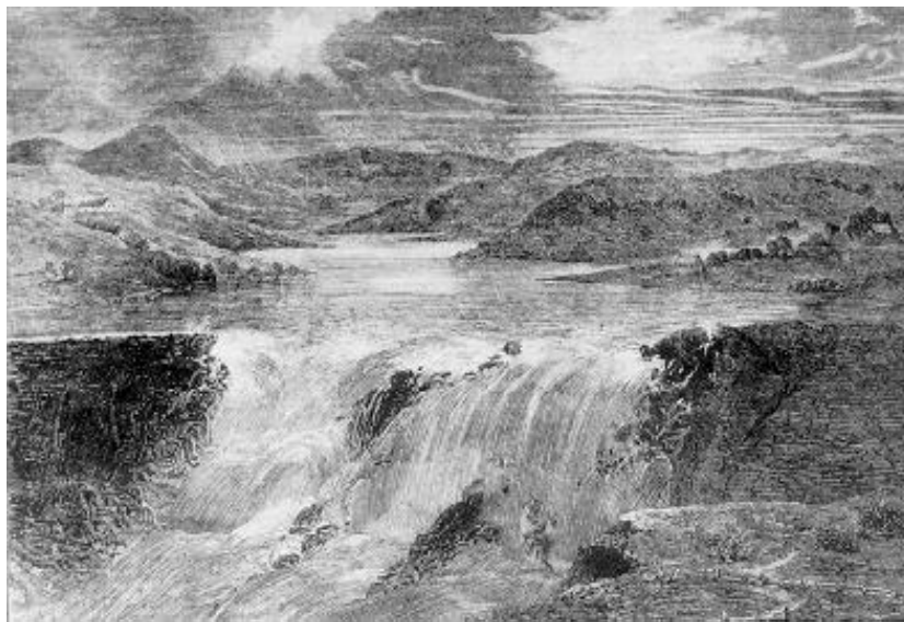
Artist's impression of the Dale Dyke Dam collapse of 1864. [Michael Armitage collection]
