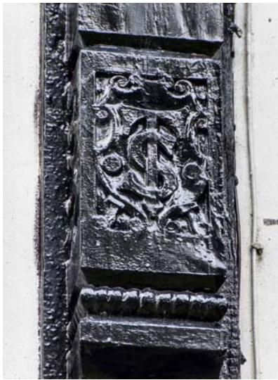
The Thomas Shaw motif carved into the decorative surround of the mock Tudor frontage. [David JW Harrison]
