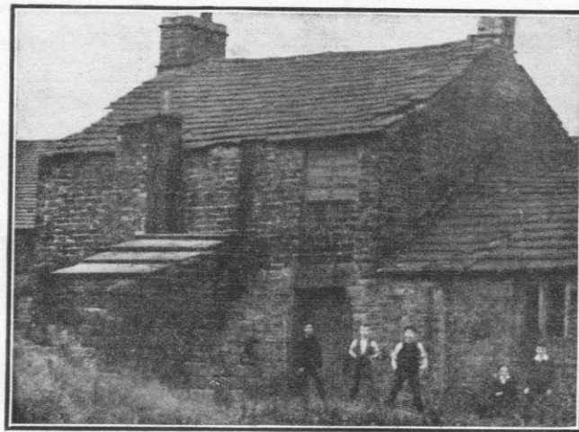
Building in which First Service was held and Sunday School Established.
