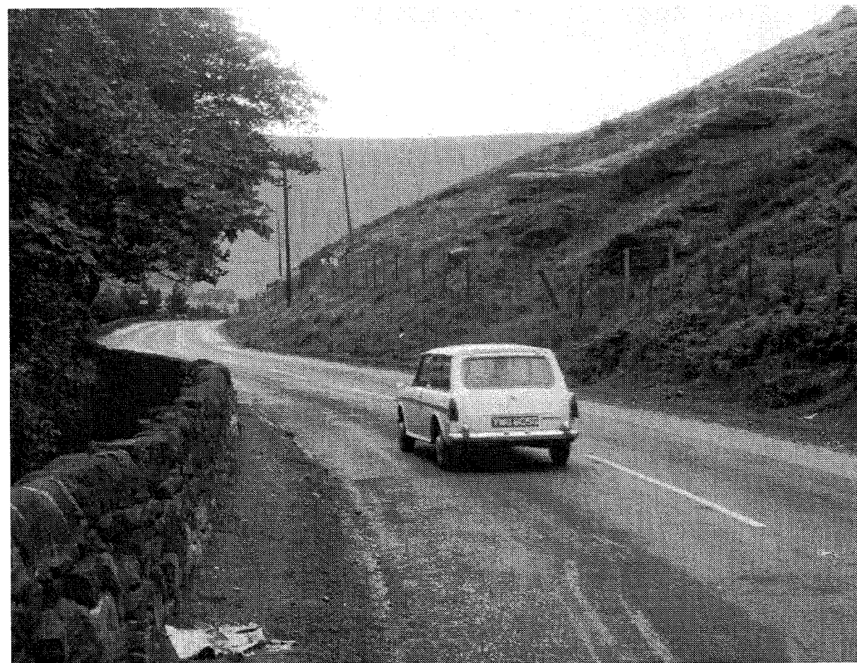
Pill Boxes on the A635 at Greenfield (Copyright of Oldham Local Studies and Archives)
