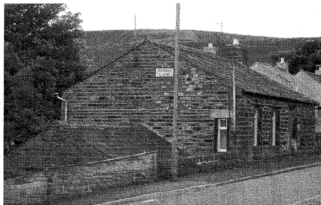
Denshaw Toll House (Huddersfield & New Hey)
