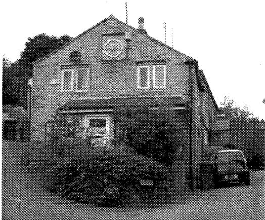
Tamewater Toll House (Branch of Oldham & Standedge)
