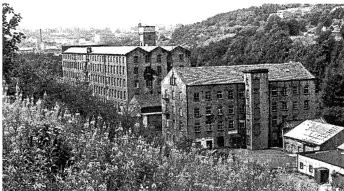
Whetley Mills, Bradford, Yorkshire. A worsted mill with spinning mill (left), warehouse (right) and single storey combing shed (foreground)
