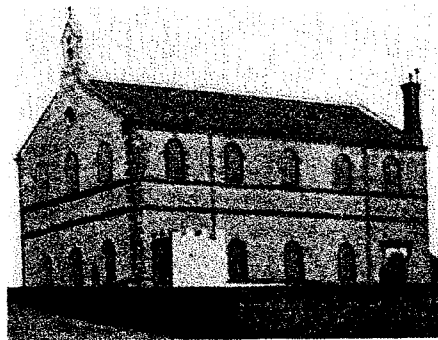
Cover illustration: St Anne's Lydgate before it lost its cupola in 1899. The photograph above shows the church without its cupola but before rebuilding commenced in 1908.
